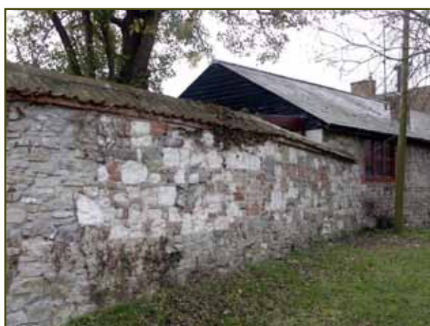
Figure 25 Tile capped walls
